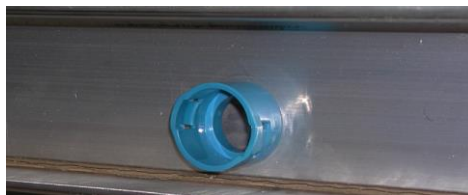
Figure 3: Conduit Hole in Scale Frame
